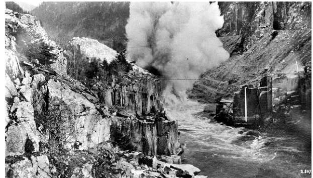
Figure 7: Detail of historical image from the table, "Clearing Hell's Gate Rockslide, Fraser River ca. 1916" (Courtesy Vancouver Public Library)
